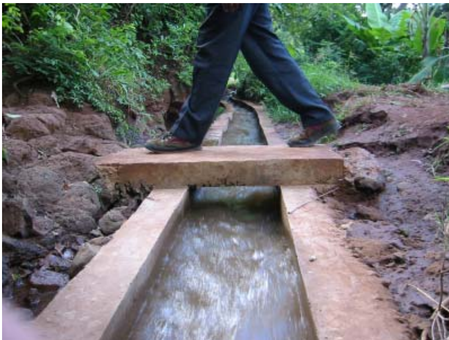
Improved traditional canal; Nganjoni irrigation scheme
